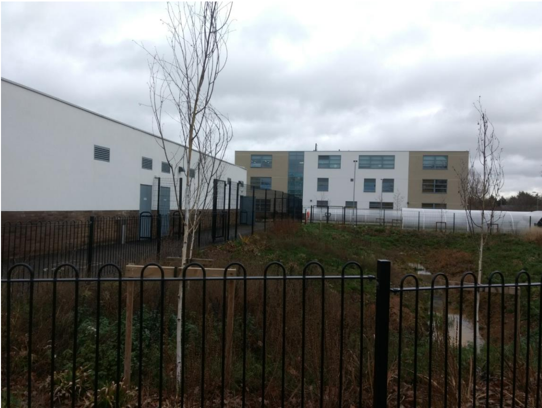
View of front elevation of Sports Block and west elevation of School Block
