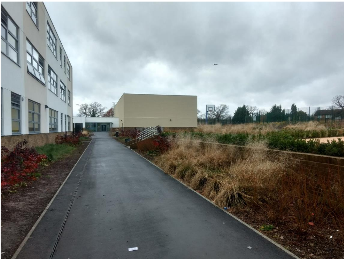
View from north elevation of teaching block looking west to sports block
